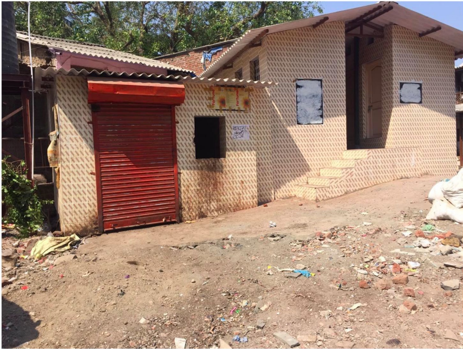
Figure 4. After the clean up drive and construction of closed garbage disposal unit.
